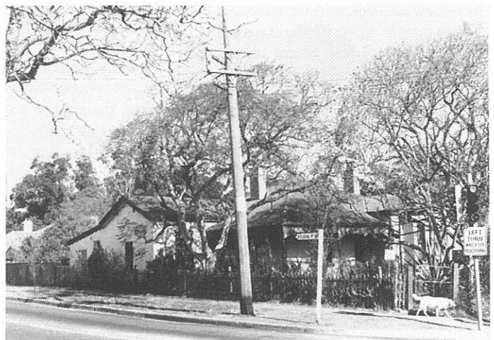
'Hope' corner of Kissing Point Road - Photo: KHS, 1971
