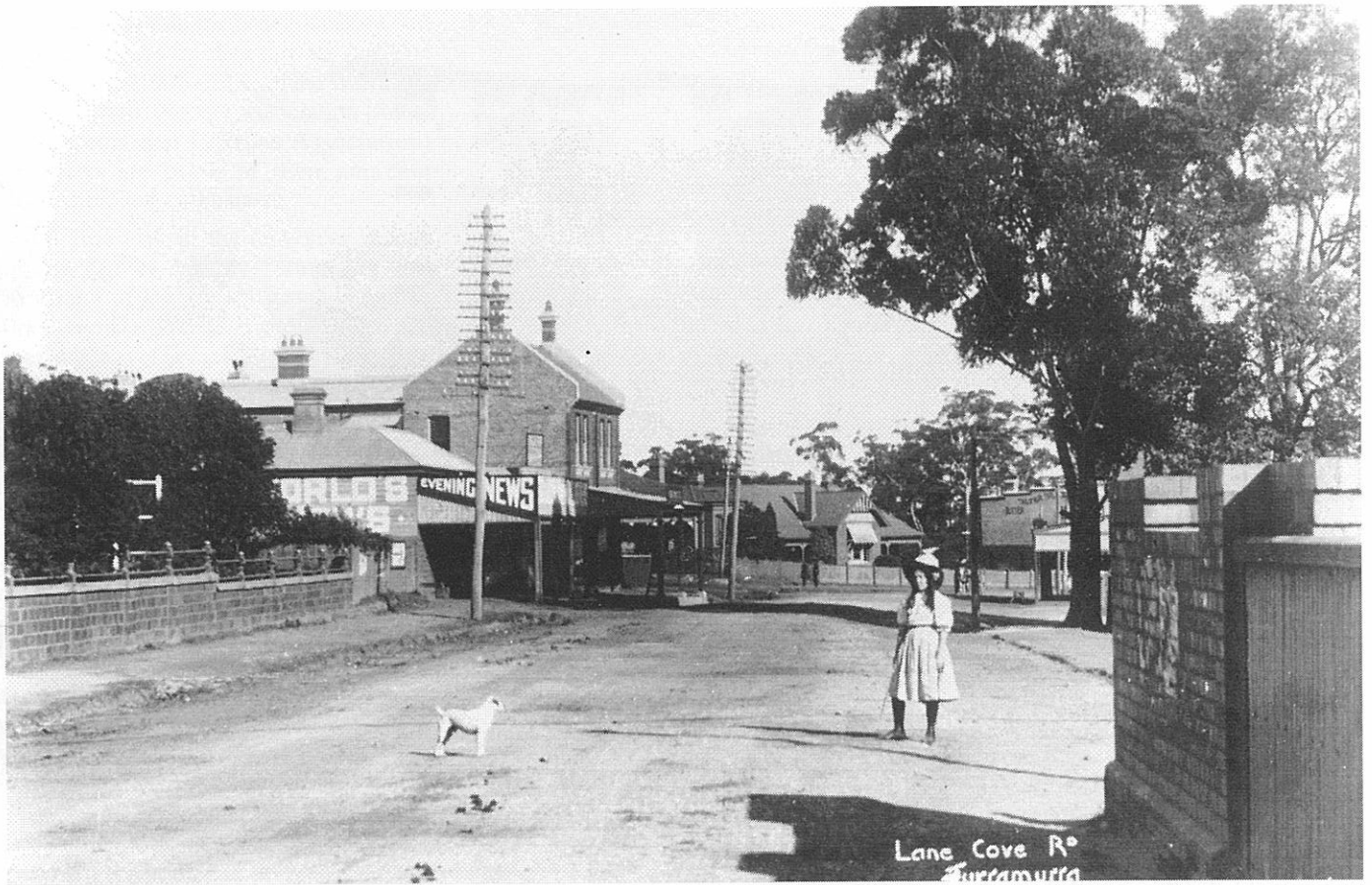
Top photo: Lane Cove Road, Turrumurra looking north from railway bridge - the two storey shops are still standing - SRA, KHS Collection
