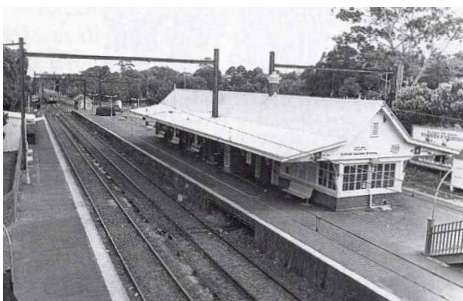
Gordon Station looking south, 1990 (note switching gear now enclosed at northern end of waiting room)
