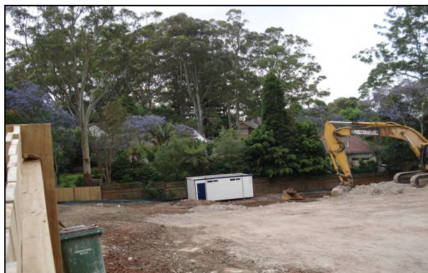
As sites are cumulatively cleared, the very basis for fragile Urban Forest ie. rich soils and seed-bank, is excavated and removed forever by improper planning.
