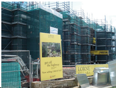
Killara - units under construction
