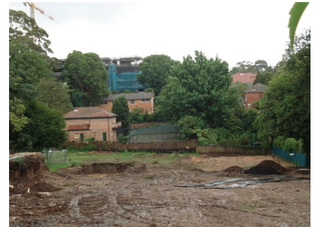
Killara-unit site cleared
