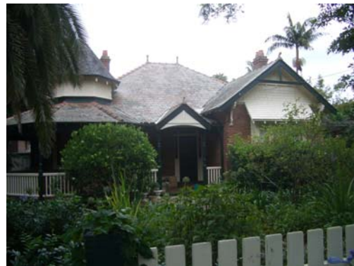
Gordon Cecil St heritage listed item Adjoining 5 storeys National Trust UCA 12
